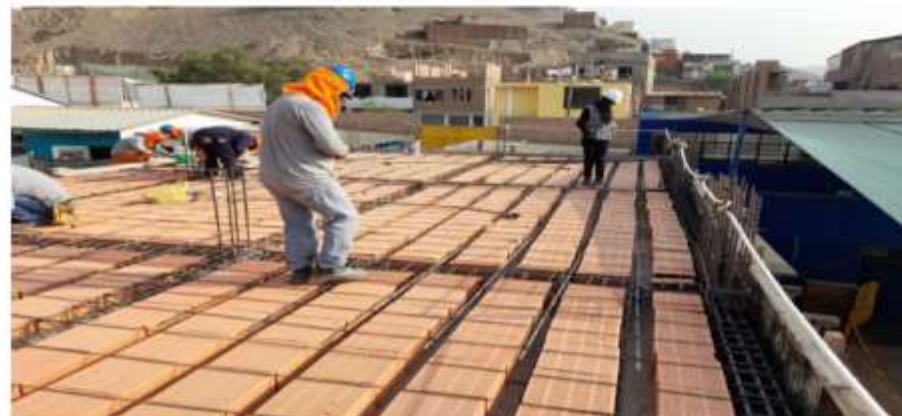
I.E. Nº5180 ABRAHAM VALDELOMAR – SECTOR LADERAS S/ 348,497.00
